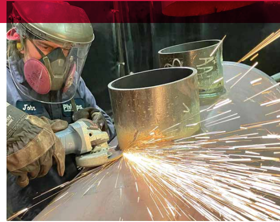
Weld blending on a stainless pressure tank with a Tiger Ceramic grinding wheel.
