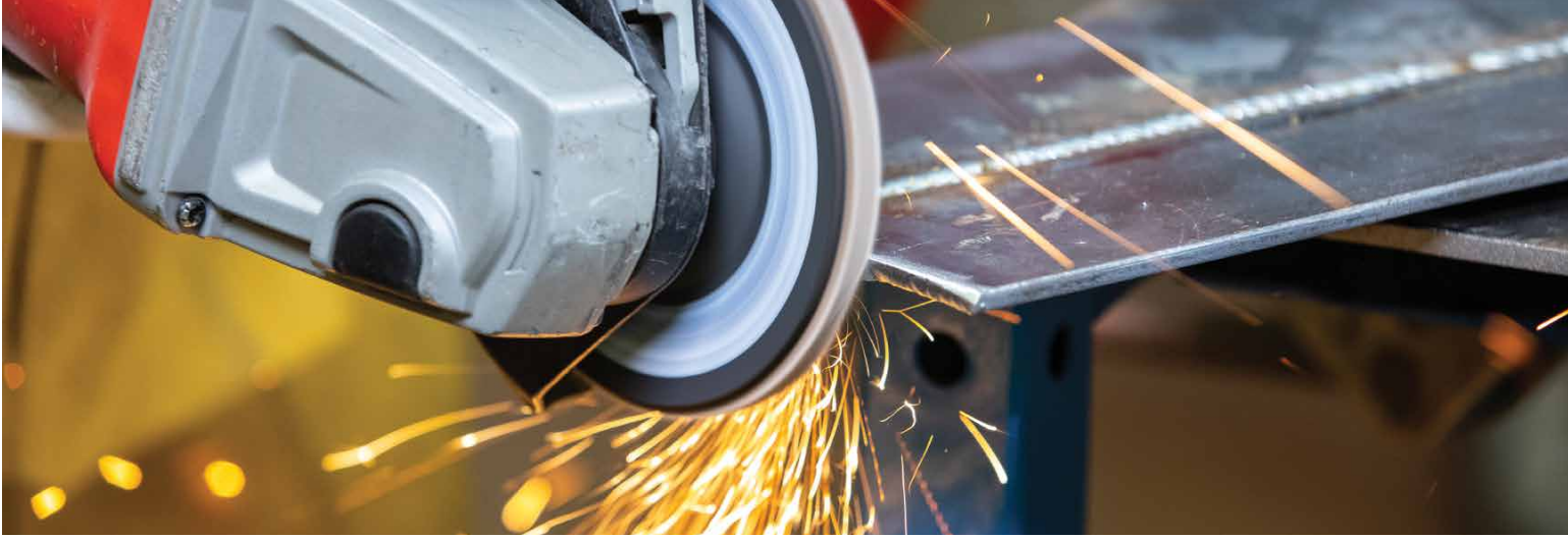
Tiger Paw grinding the edge of a torch-cut steel plate.
