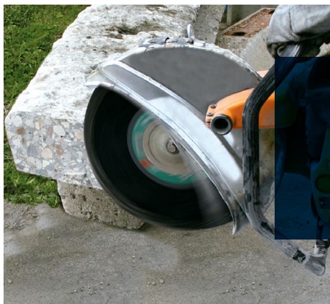
Metalynx PRO Stone wheel cutting a curb.
