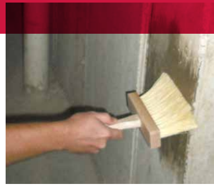
Applying waterproofing material with a masonry brush.
