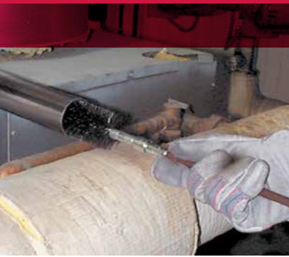
Cleaning boiler pipes with a flue brush.
